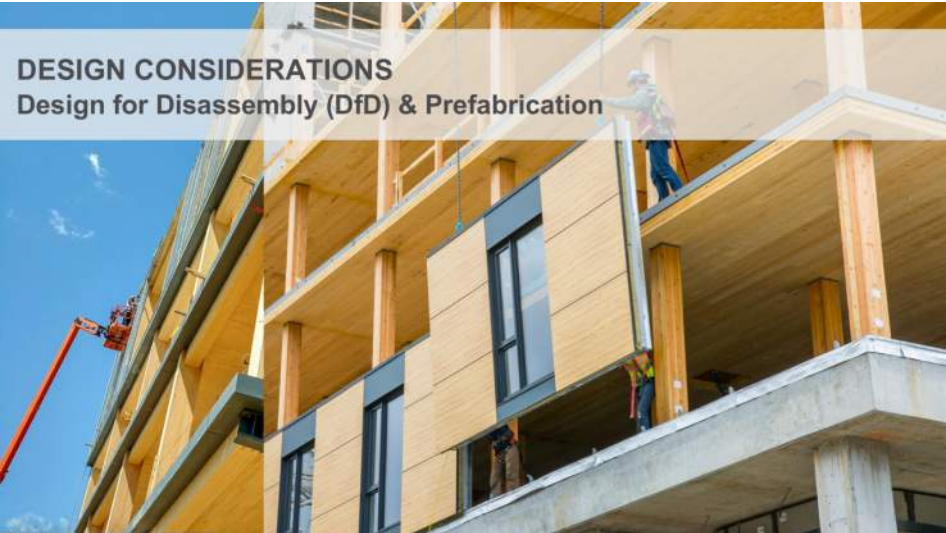
Figure 25. Prefabricated wall panel construction.
